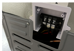
New Wiring System
