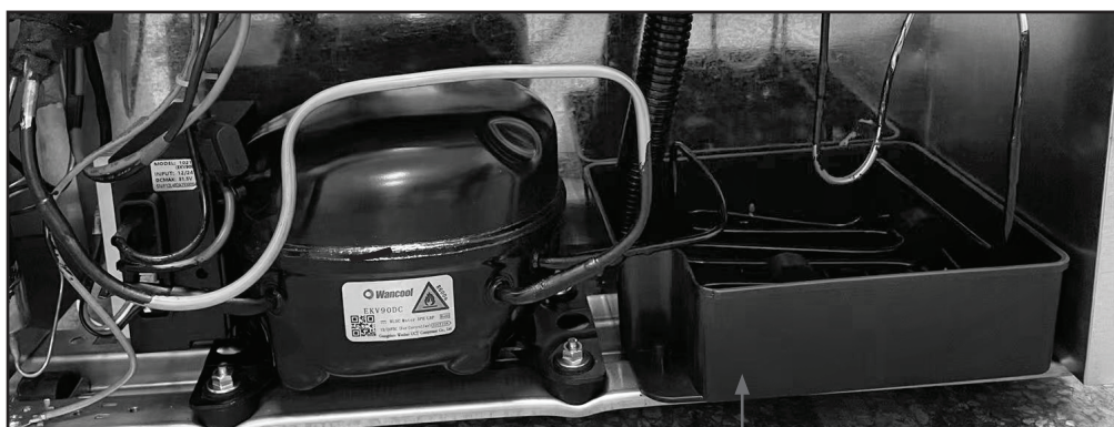
• water catch basin
